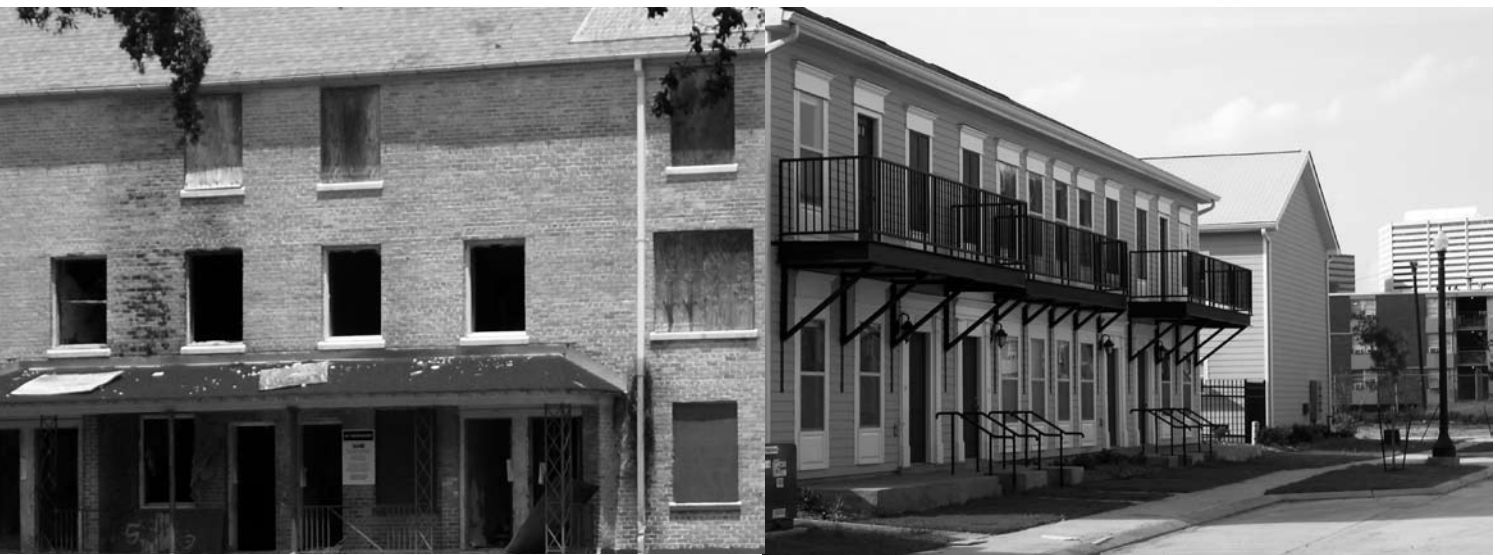
From the 1940s to now, dilapidated units stand as idle reminders of failed housing projects (left). Mixed income developments remain empty (right).
