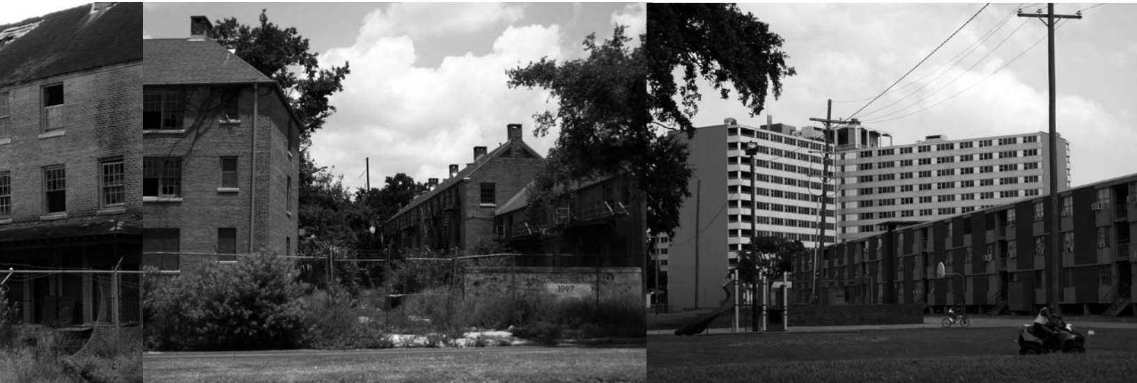
Weeds and broken fences surround the empty projects (left, center). Few children play alongside the Guste projects (right).
